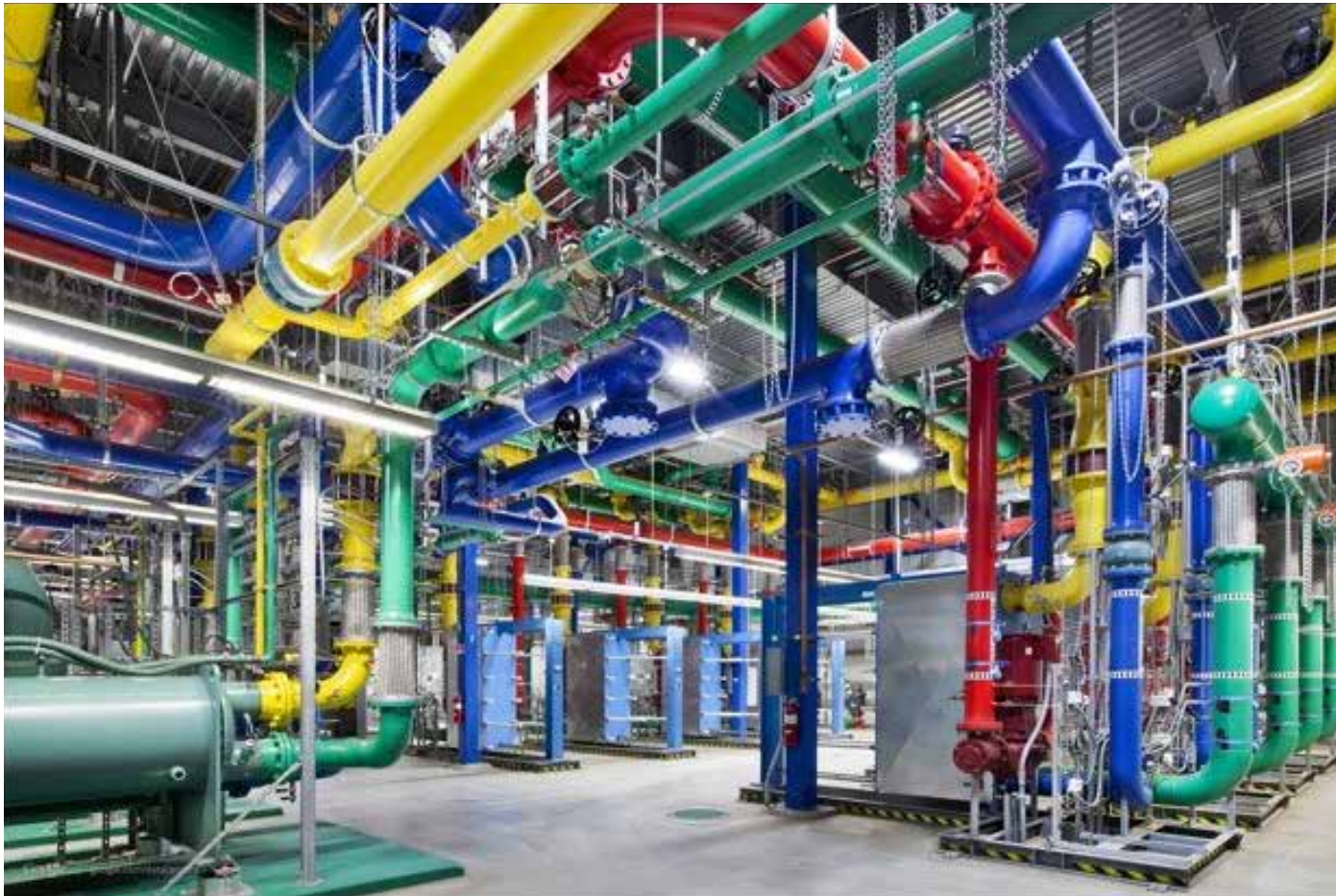
Fig. 7: The tubes of the Internet. The water cooling system in the Google data center in The Dalles, Oregon. Source: Connie Zhou for Google. 2012.
